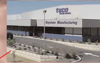
Perth Western Australia Keystone Slurry Products
